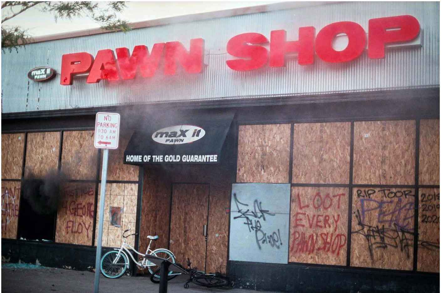
May 28: A looted pawn shop east of the Third Precinct on Lake Street about to catch fire. The story spread that the previous night, the owner had shot and killed someone.
